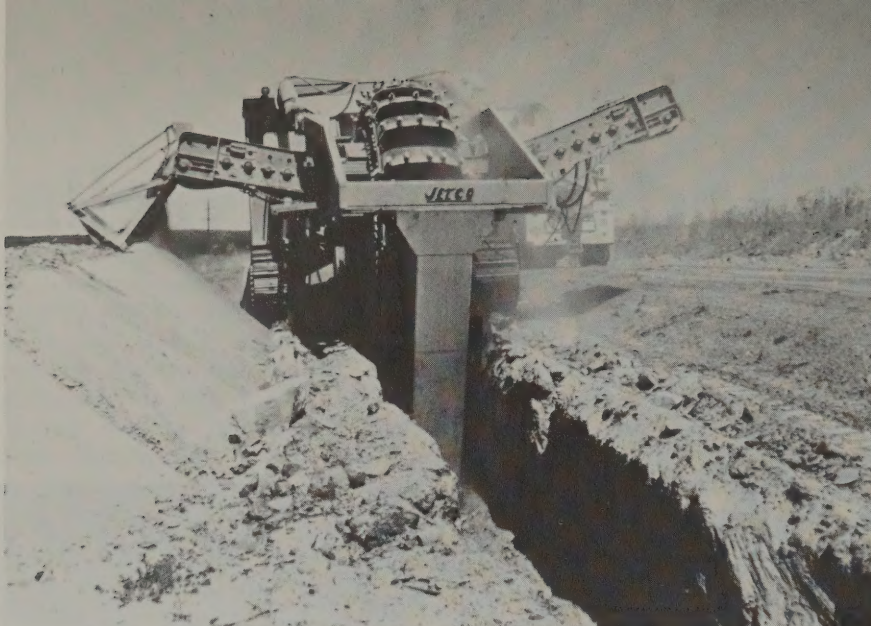
Pipeline trenchers such as this minimize surface disturbance.
